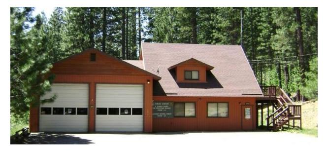
El Dorado County Fire Station 16 is located at 13275 US Highway 50 in Kyburz CA. This is a 2 story, 3,000 sq. ft. building, last updated in 1990. The current composition roof has reached the end of its service life and the District is looking for bids for replacement. The project would include:
